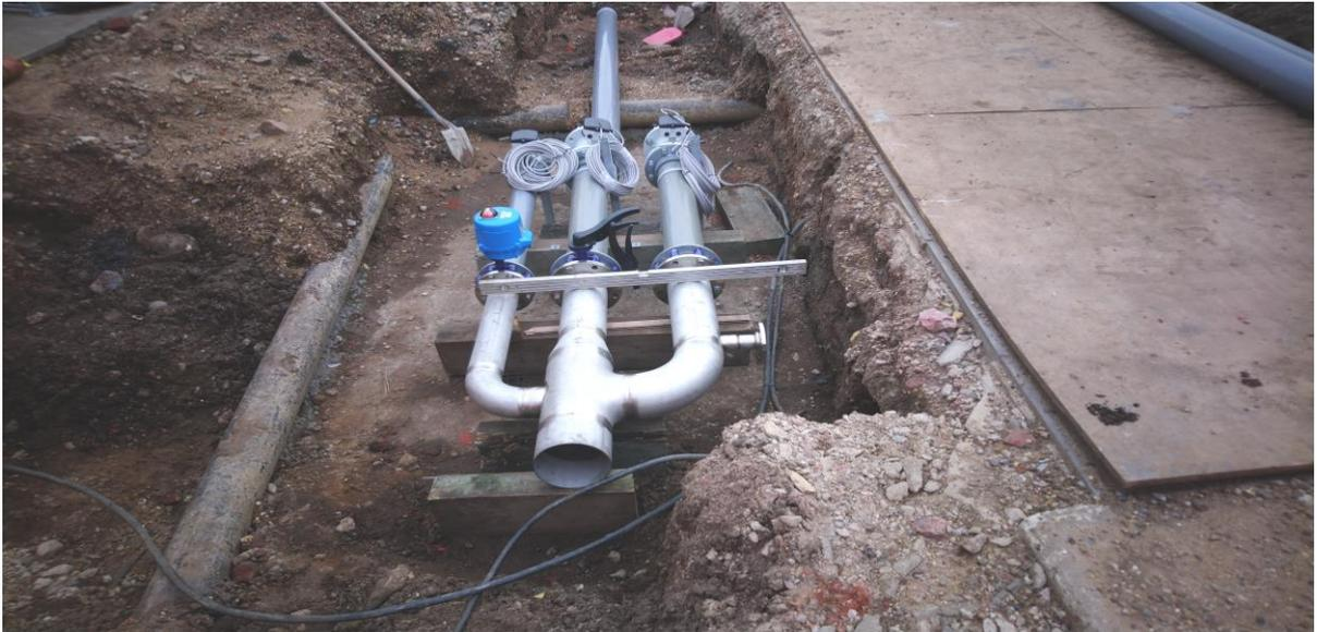
New stainless steel and ABS industrial plastic pipework is being installed below the ground to provide enhanced filtration of the water. Once finished this pipework will be hidden from view. The new system includes automatic valves to keep the toddler pool water level constant and flow monitoring equipment to be sure the filtration system works to its greatest efficiency.
