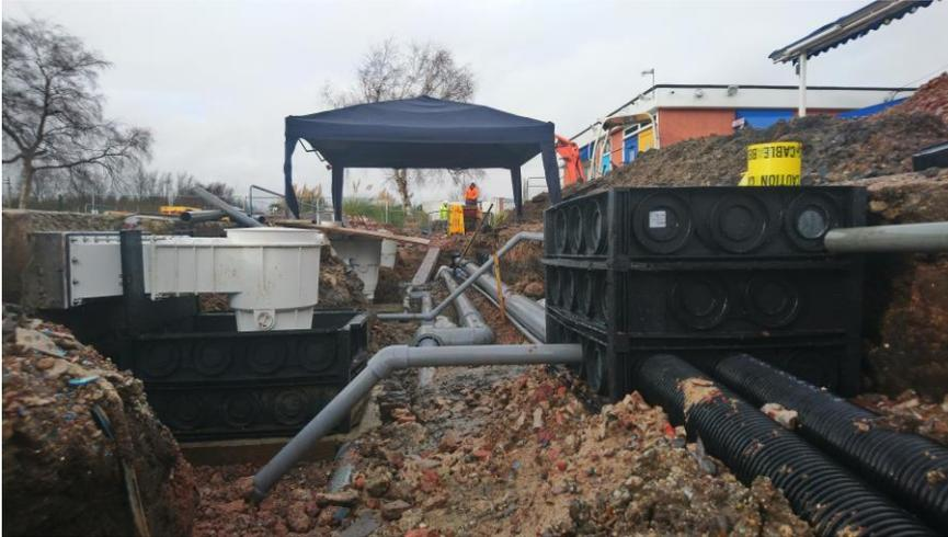
The complex pipework system includes eight new high capacity surface skimmers that will improve the water quality for the swimmers.
