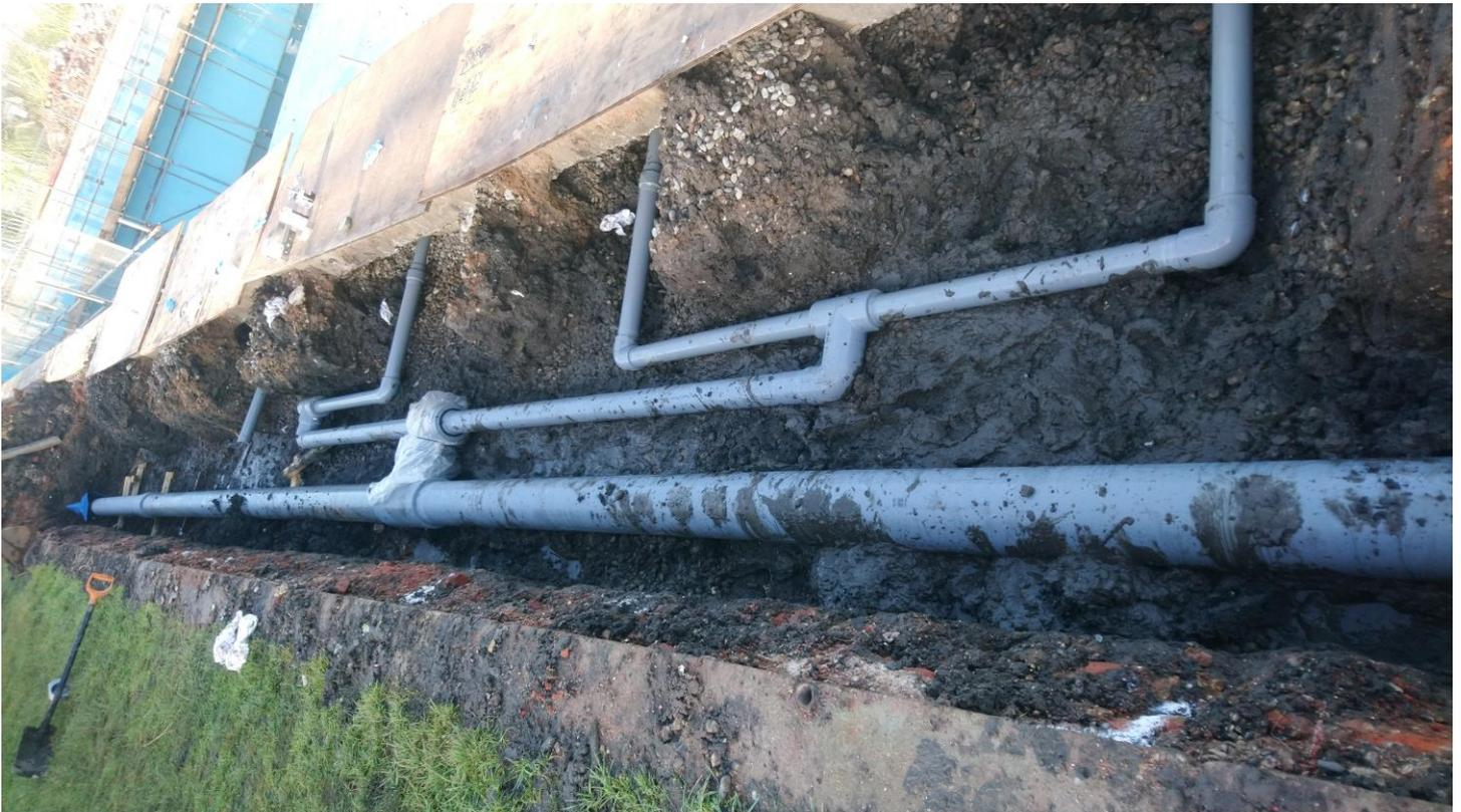
New return pipework is starting to take shape with a total twelve new pool return ports. The new pipework is made from heavy duty industrial plastic that will give the pool at least another 60 years of service to the community. This new pipework will enable the entire one million litres of water to be pumped through the filtration system more efficiently. All of this pipework will be hidden once more as the project proceeds towards completion
